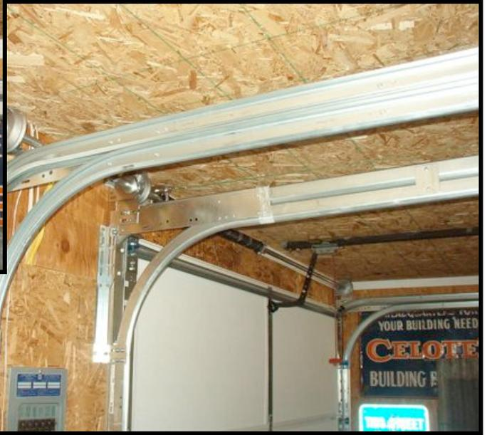
The trick to this install was the low clearance tracks that Kevin sourced to make the doors fit into the low ceiling height that I have in the barn. If you notice to the right photo, the tracks are a dual set up to make the geometry of the door lift function as it should. Compare this to your standard garage door and you will see the obvious difference. Who would have known? Not me!
