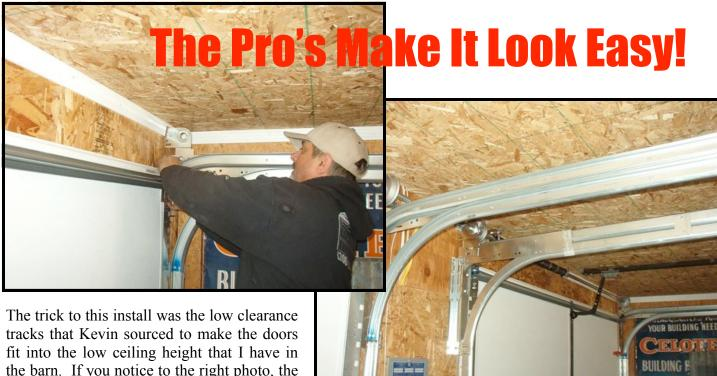
The trick to this install was the low clearance tracks that Kevin sourced to make the doors fit into the low ceiling height that I have in the barn. If you notice to the right photo, the tracks are a dual set up to make the geometry of the door lift function as it should. Compare this to your standard garage door and you will see the obvious difference. Who would have known? Not me!
