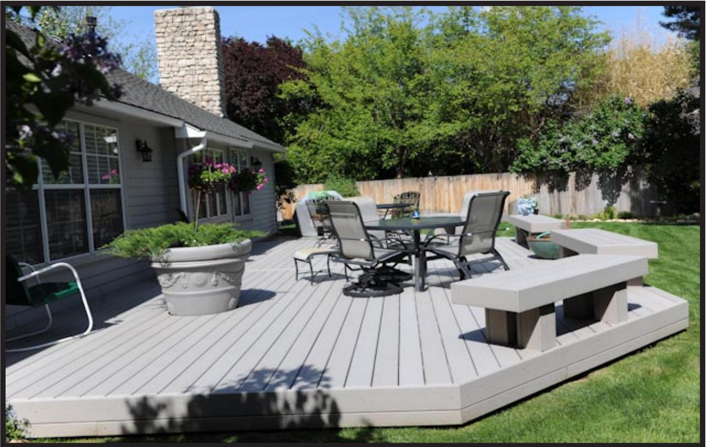
Day two we were able to install most of the new decking and on day three we finished up the deck. Day four we installed the new "Floating" skirt, and built the new benches. We also framed in a hole in the deck and recessed the huge potted bushes into the deck rather than setting the pot on the deck. This will allow for drainage and will not create a sag in the deck or stains from the pot.
