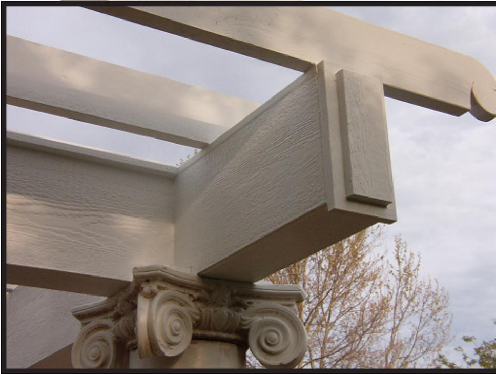
The beams are 24' long with 66" connections between them. They are screwed to the top of the 4x4 posts which extend 3/4" beyond the top of the columns.
